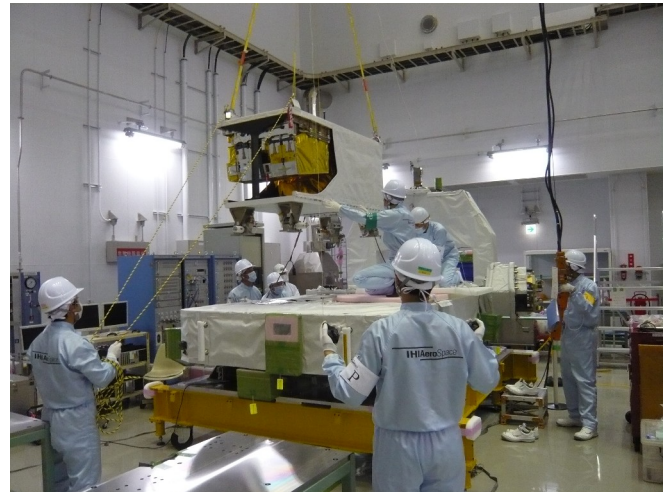
Figure 2: HREP (with RAIDS visible) is lowered onto the Experiment Pallet in a clean room at Tanegashima Space Center, Japan in May, 2009.
